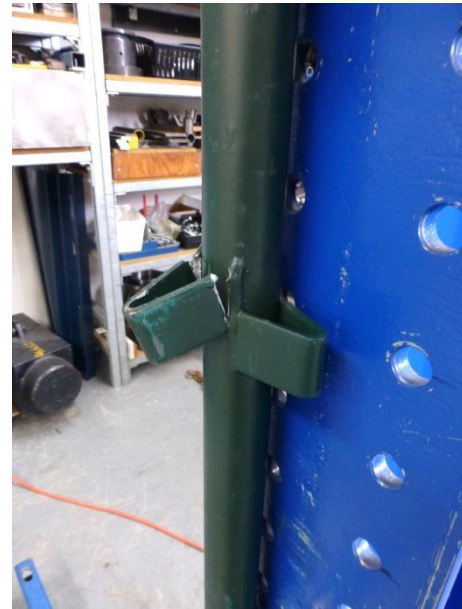
FIG.6 FAILURE OF V-PRESSING
